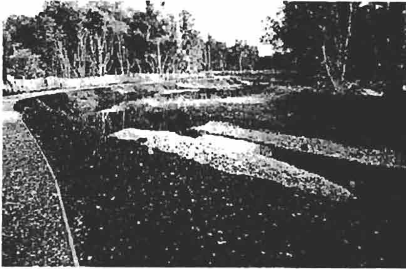
Figure 11.3 A riffle reinstated in a river in south-central England (courtesy of S. Reed)
