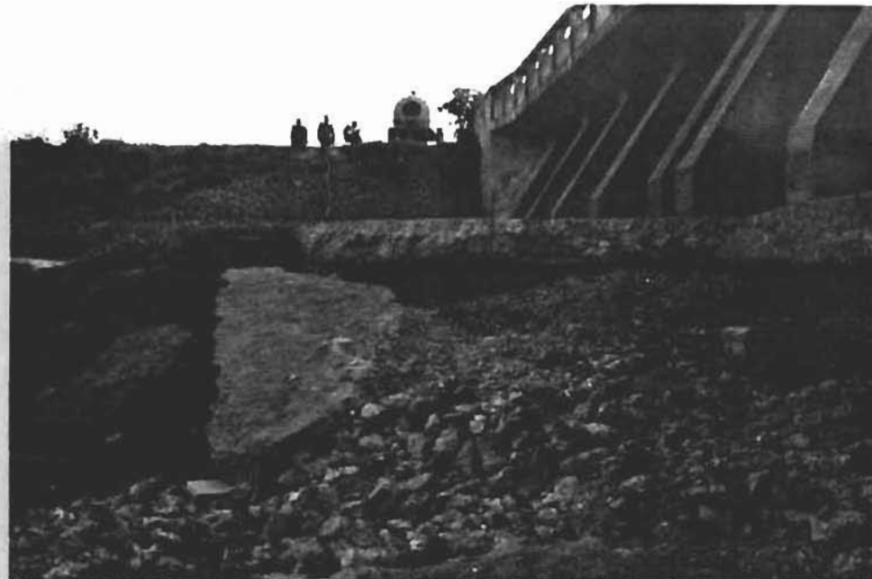
Photograph 3: The concrete apron
