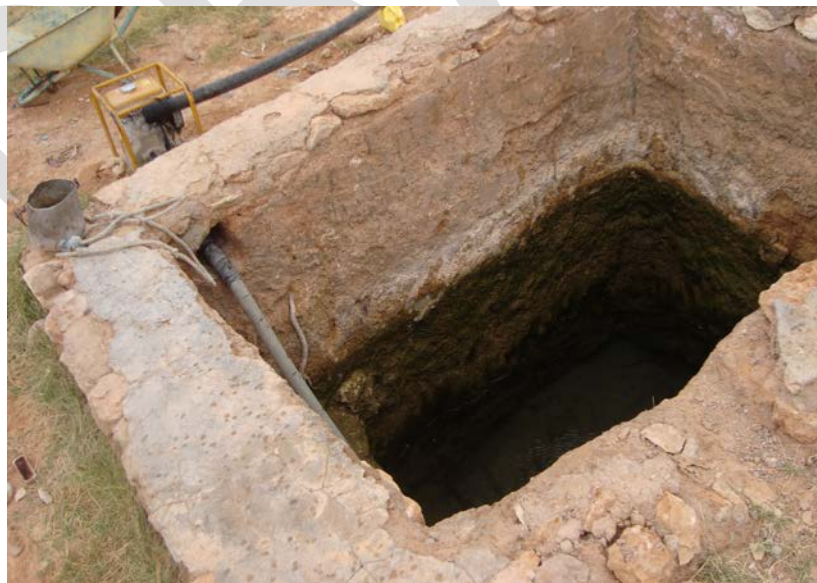
Photo 8: Shallow well with water in Irrigated agricultural near Garowe. (notice the diesel pump for irrigation)
