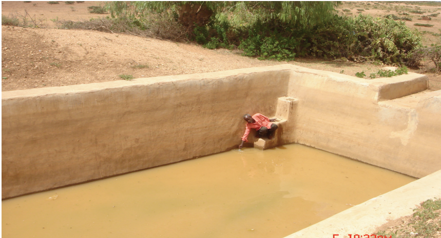
Figure 4.1 Rectangular berkad with concrete wall
