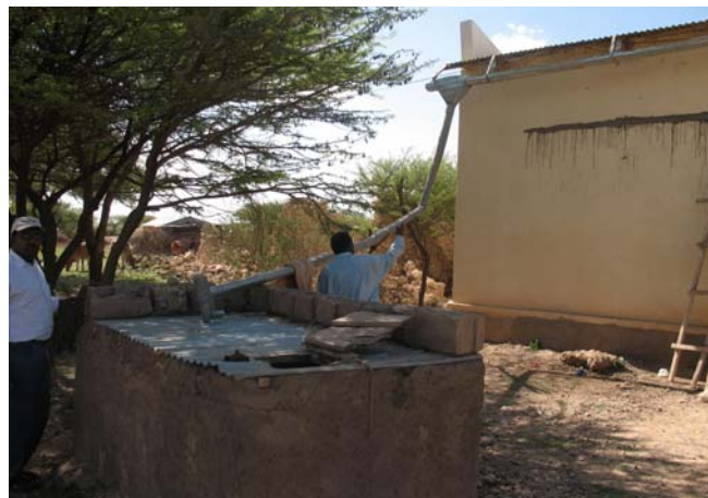
Plate 11: A Berkad guri showing the roof runoff harvesting components
