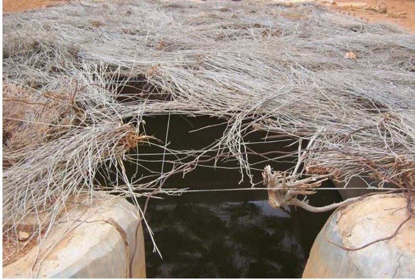
Plate 10: Mitigating evaporation losses from berkads using grass covers
