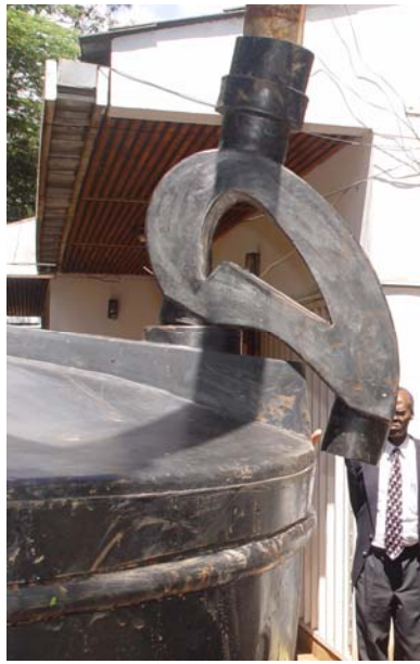
Plate 15: Manual foul flush mechanism
