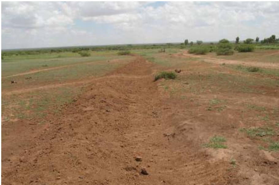
Plate 5: Runoff conveyance channel during construction
