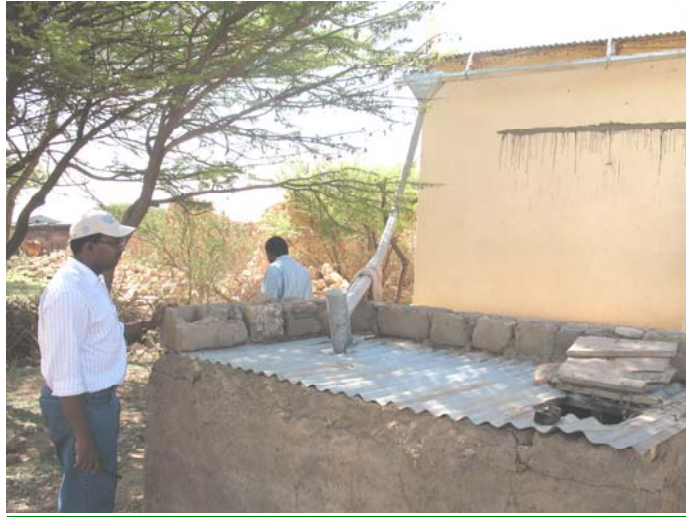
Plate 2: A typical Berkad guri depicting the catchment, conveyance and storage components
