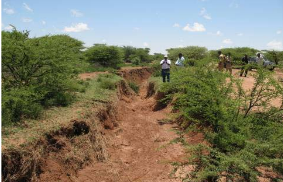
Plate 6: Runoff conveyance channel in north-west Somalia after having developed into a gully and conveying a lot of silt to the pond
