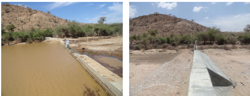
Figure 14: Sand dam after flood and dry, filled with sediment
