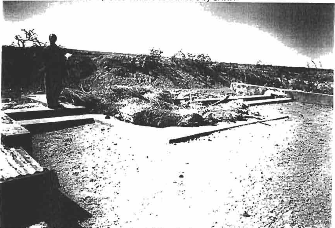
Plate 10: Improved inlet channel and silt trap for improved berkad - SAWA
