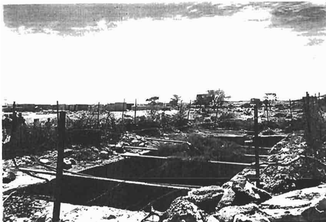
Plate 11: One of the oldest berkads – Constructed 1 1959 (Hiriro village)
