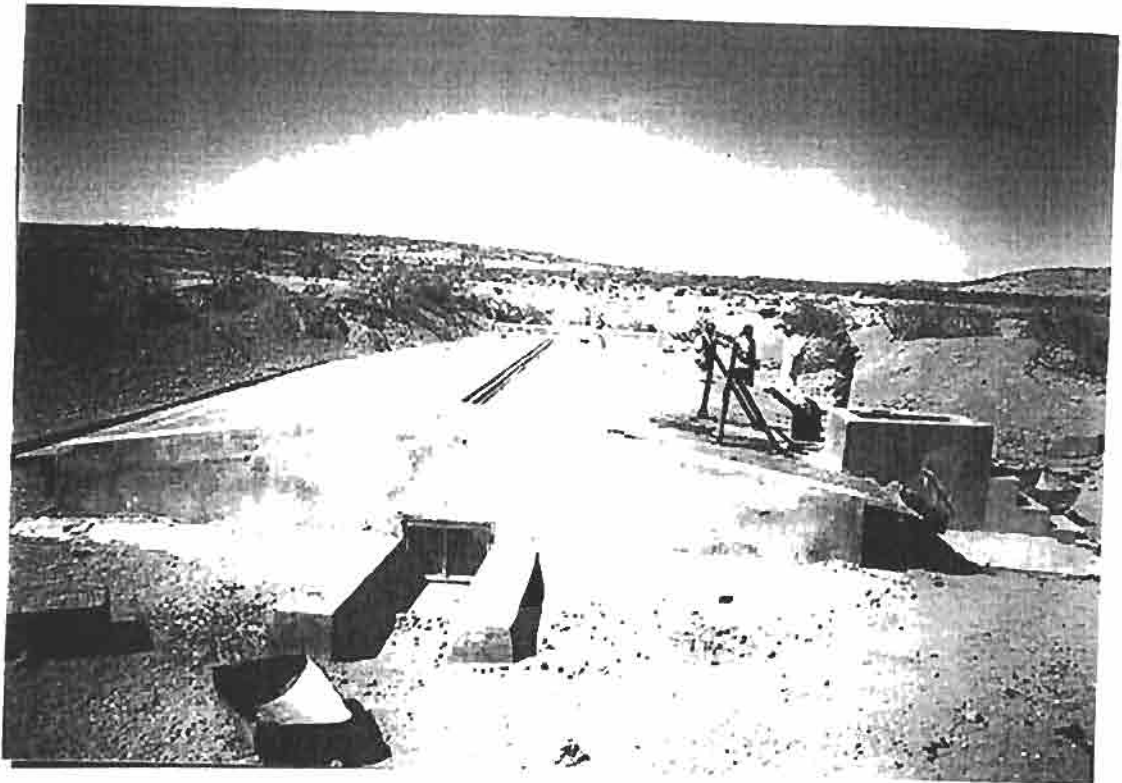
Plate 9: Improved berkads constructed by SAWA
