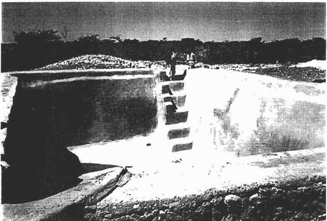
Plate 6: Berkad repaired by Oxfam-GB in Qudah village, Galbeed area, Somaliland
