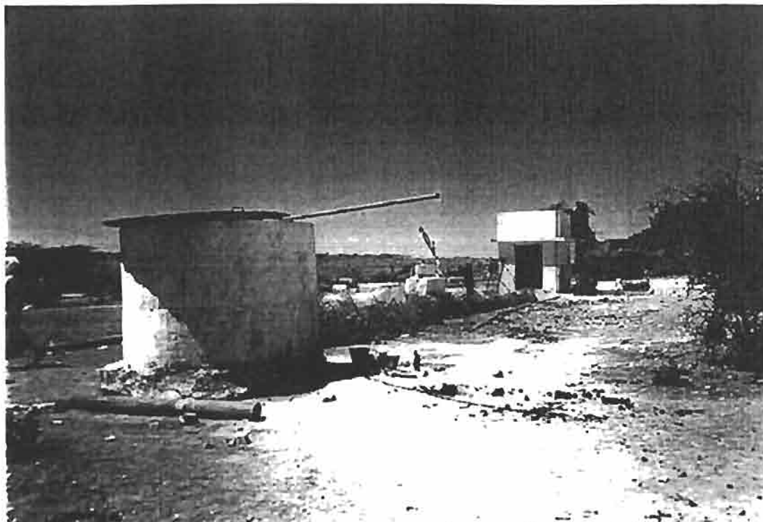
Plate 3 : Borehole with pump house and small tank, Adinsoone village, Gardo District
